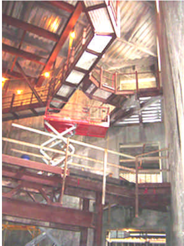
Figure 6: AlloSphere construction status as of Summer, 2005, showing the bridge across the bottom and “halo” ring truss at the top
