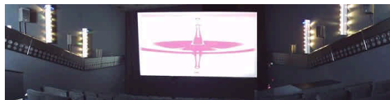
Figure 14: 198-channel cinema in Ilmenau, Germany; along the walls are the closely spaced loudspeakers for wavefield synthesis.
